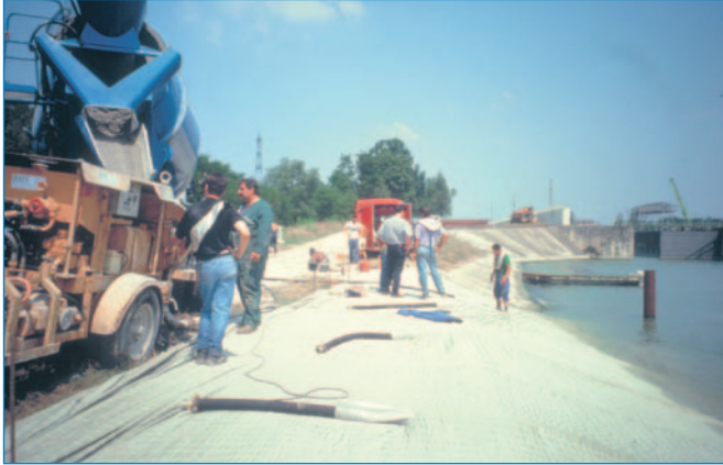
Filling the mattress using a concrete pump
