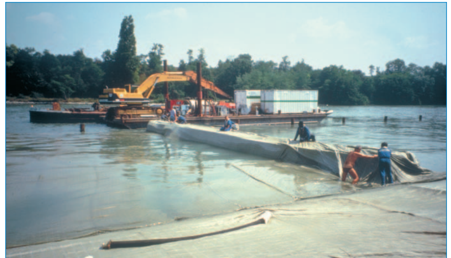
Captions: Placing a panel on the barge
