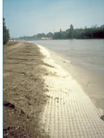
The restored canal access after the mattress installation
