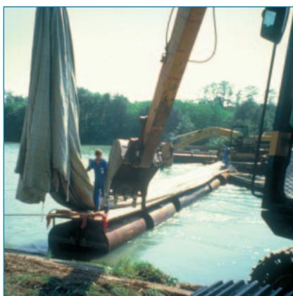
Placing a panel on the barge for installation
