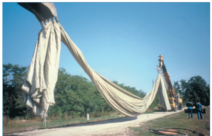
Bringing a panel onto site
